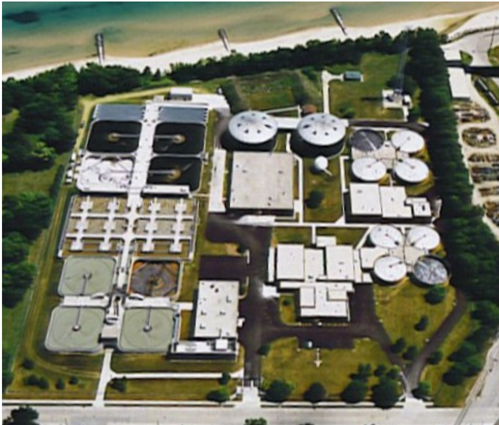
Figure 1: Aerial View of the Sheboygan Wastewater Treatment Plant (Photo provided courtesy of Sheboygan Regional WWTP)
