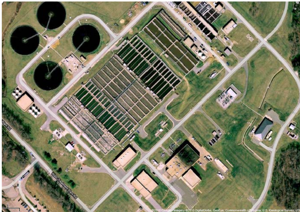
Figure 1: Washington Suburban Sanitary Commission Western Branch WWTP
