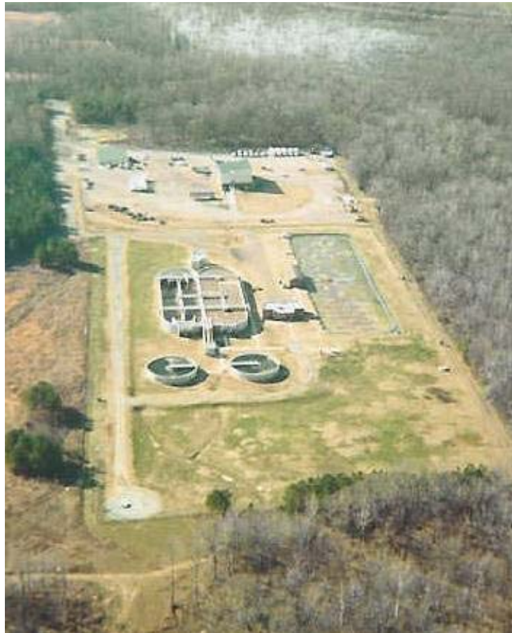
Figure 1: Aerial View of the City of Bartlett Wastewater Treatment Plant #1 (Photo provided courtesy of the City of Bartlett Wastewater Division)
