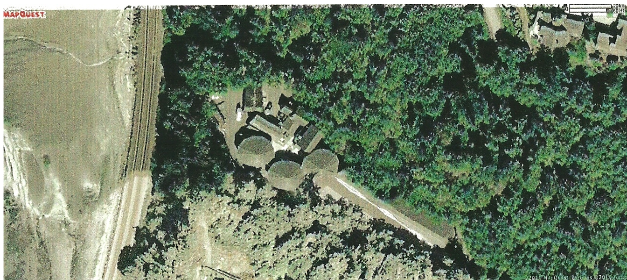
Figure 1: Aerial View of Big Gulch WWTP
