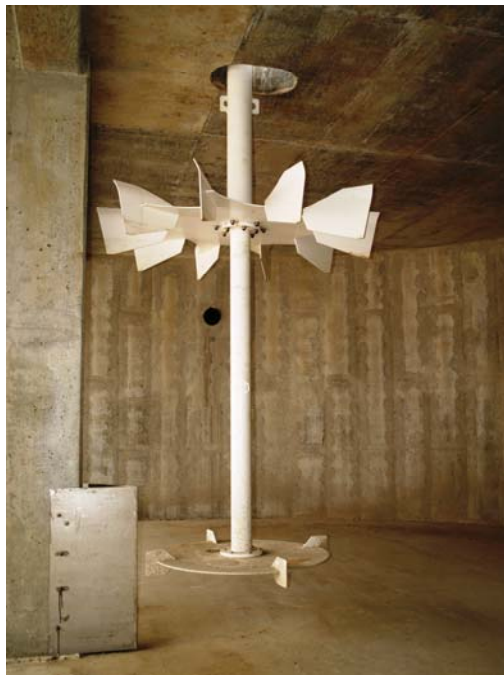
Figure 4-1. Eimco Water Technologies Carrousel ® System Excell ® Aerator II Source: Eimco Water Technologies. Used with permission.
