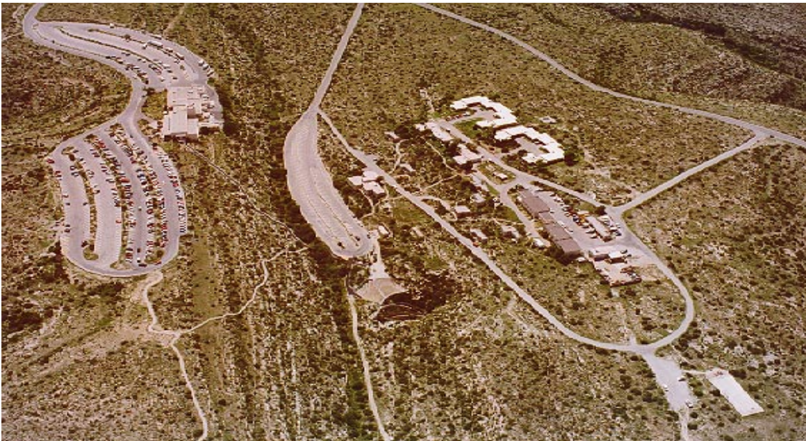
Aerial view of Carlsbad Cavern area with the NPS infrastructure built directly over the cave. The entrance is in the lower, central part of the photo. (NPS Photo)
