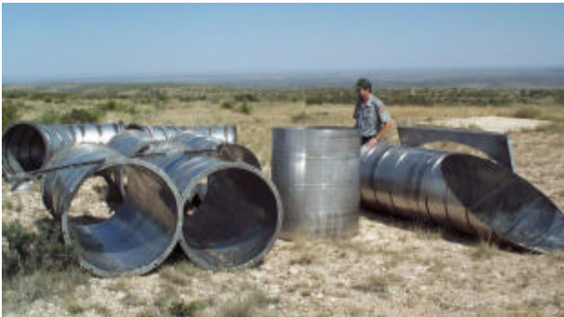
Culvert pieces awaiting transport and assembly (Stan Allison for scale). (NPS Photo by Dale Pate)
