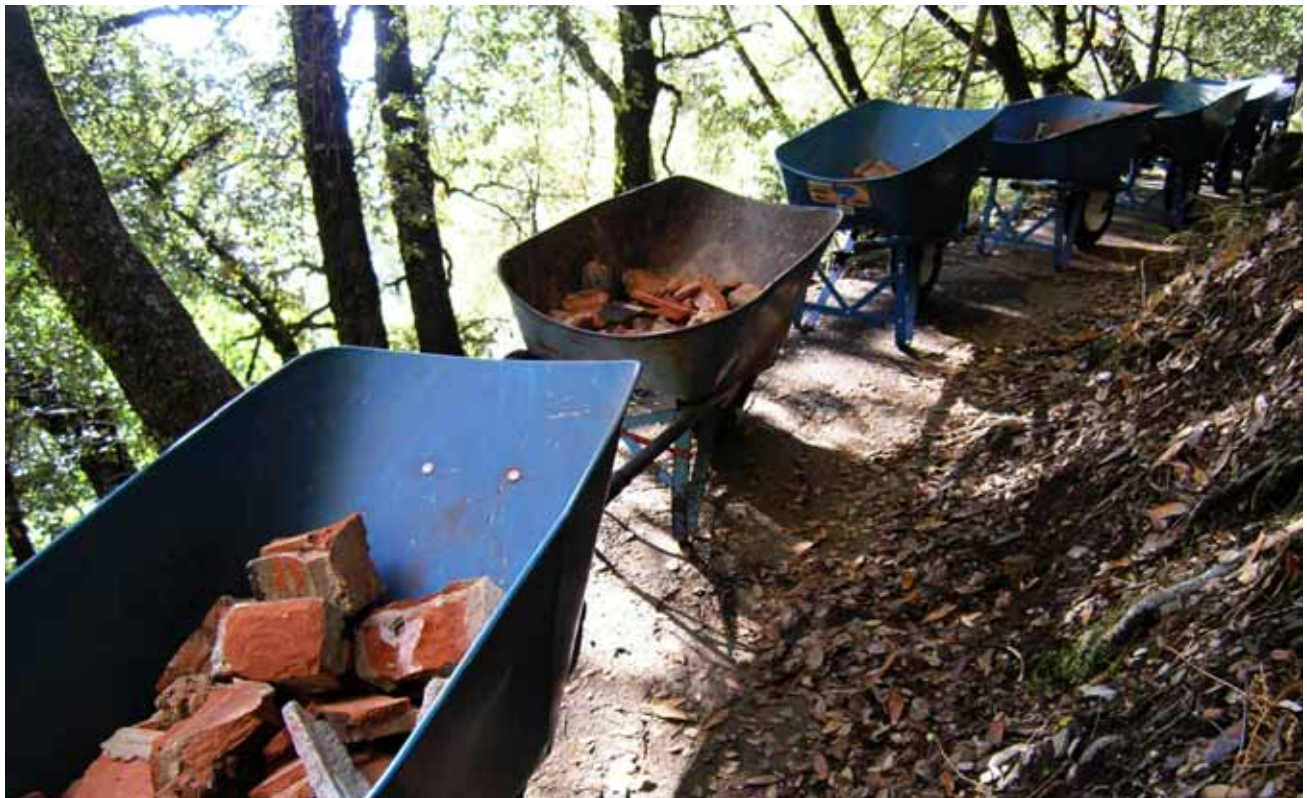
Wheel barrows were moved in groups by volunteers during the Crystal Cave Restoration. Here a "train" has developed above a set of stairs on the trail.
