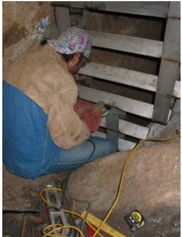
Charlie Savas of Zara Environmental welds a new gate in place on the main entrance to Soldiers Cave. Park staff hopes this gate is more bat and wildlife friendly, and more secure to help protect this delicate cave.
