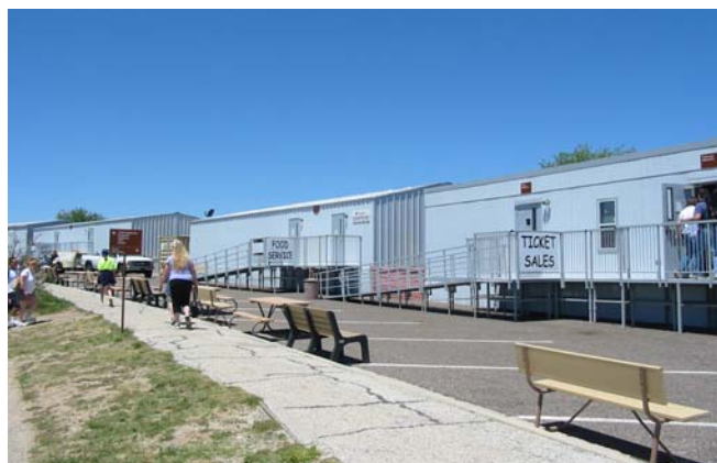
Visitor Center services at Carlsbad Caverns National Park are being conducted in these temporary trailers while the existing building is being completely remodeled.
