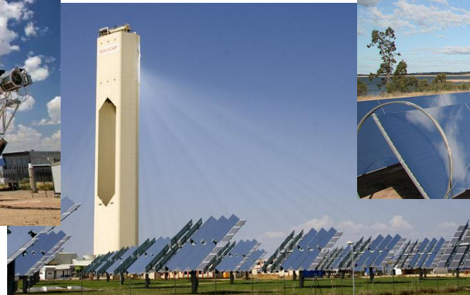
PS10 Spain, Power Tower
