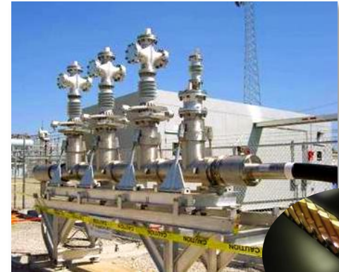
Triaxial superconducting cable installed at AEP Bixby
