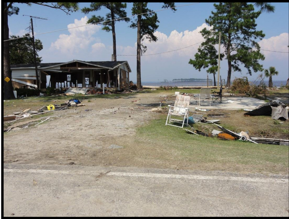
Figure. A home (right) swept off its foundation with another home (left) destroyed in Jarvis Landing
