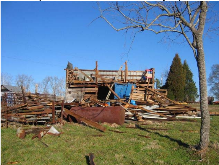
Photo 3 (Vinson Road – Barn destroyed)
