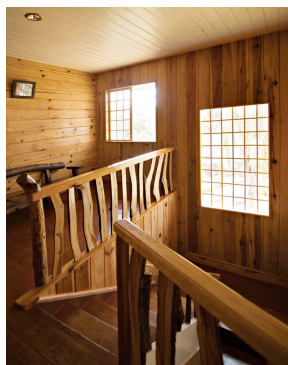
Performance software may best reflect the thermal heat capacities of mass walls (see What is a performance approach? ).
