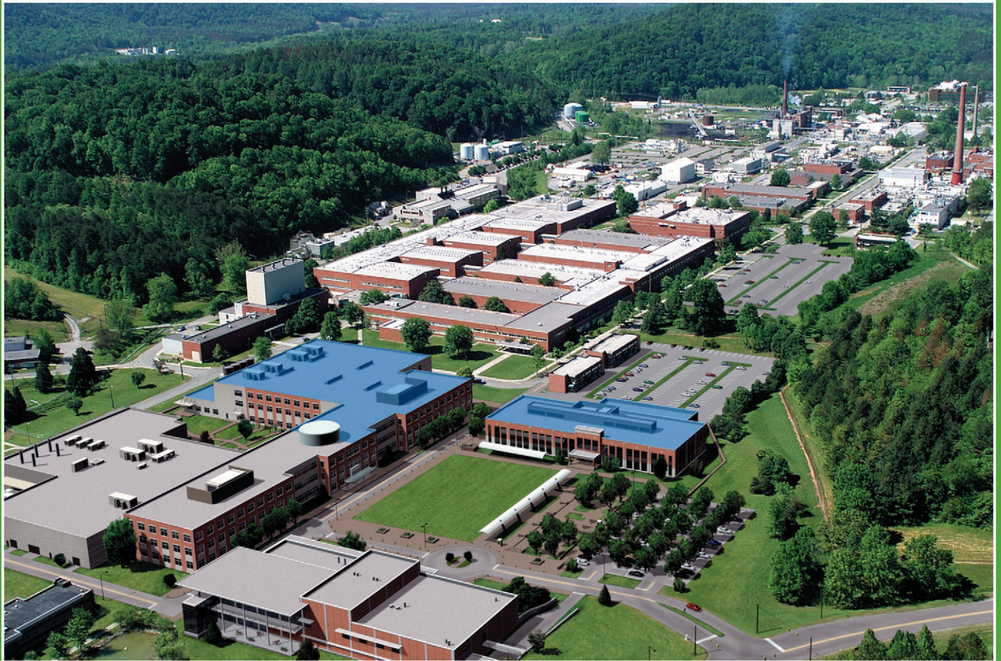
Artist's conception of the new East Campus to be constructed at ORNL by 2003. The blue overlay (not the color of the actual roofs) indicates the two buildings where computer and computational scientists from ORNL and the University of Tennessee will work. The building on the left is the privately funded Computational Sciences Building, which will house the Department of Energy's Center for Computational Sciences. The building on the right, which will be constructed using funds from the state of Tennessee, will house the ORNL-University of Tennessee Joint Institute for Computational Sciences. The buildings behind these new buildings (center and top right) are part of the existing ORNL facility. Rendering by John K. Jordan.
