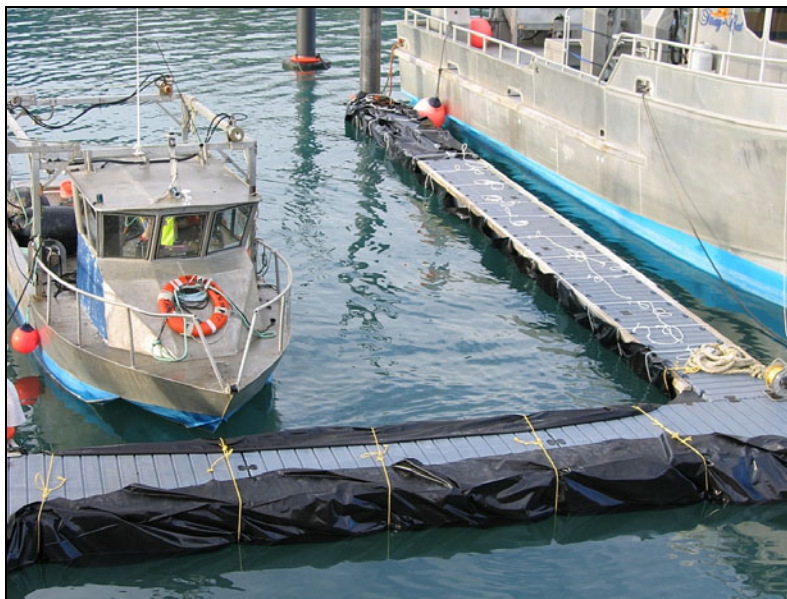
Figure 6. Jetties/pontoons were treated using the set-n-forget plastic encapsulation method or had ~ 5% acetic acid added to accelerate the treatment process.
