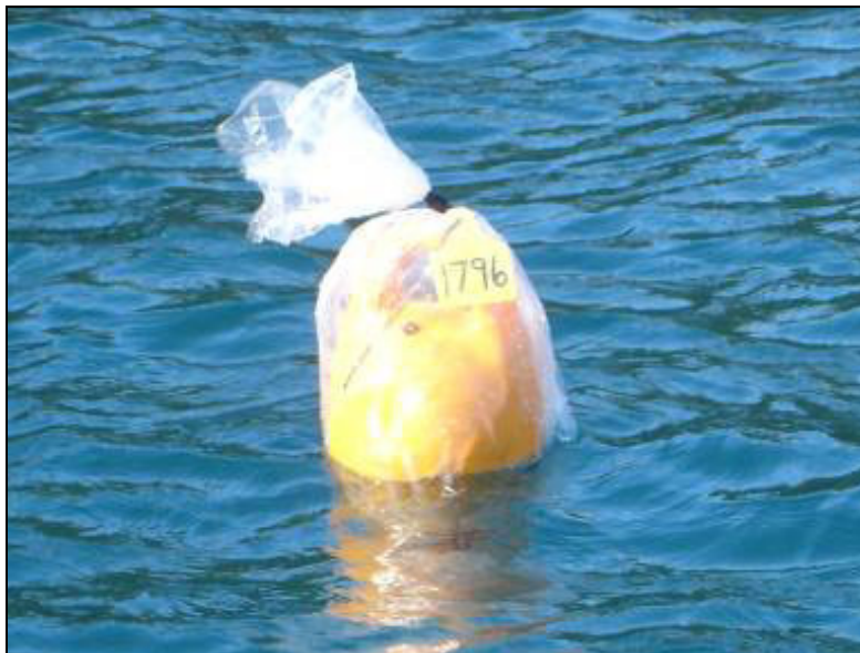
Figure 8. Vessel moorings treated using an in situ plastic set-n-forget encapsulation technique.
