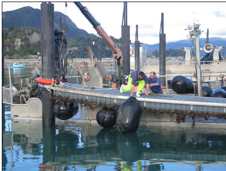
Figure 5. Lifting jetties/pontoons to treat D. vexillum .
