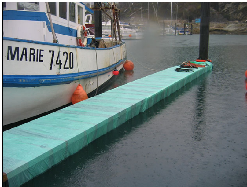
Figure 7. Some jetties/pontoons were wrapped with Donagheys plastic balage wrap, similar to the methods used to wrap vertical wharf piles.
