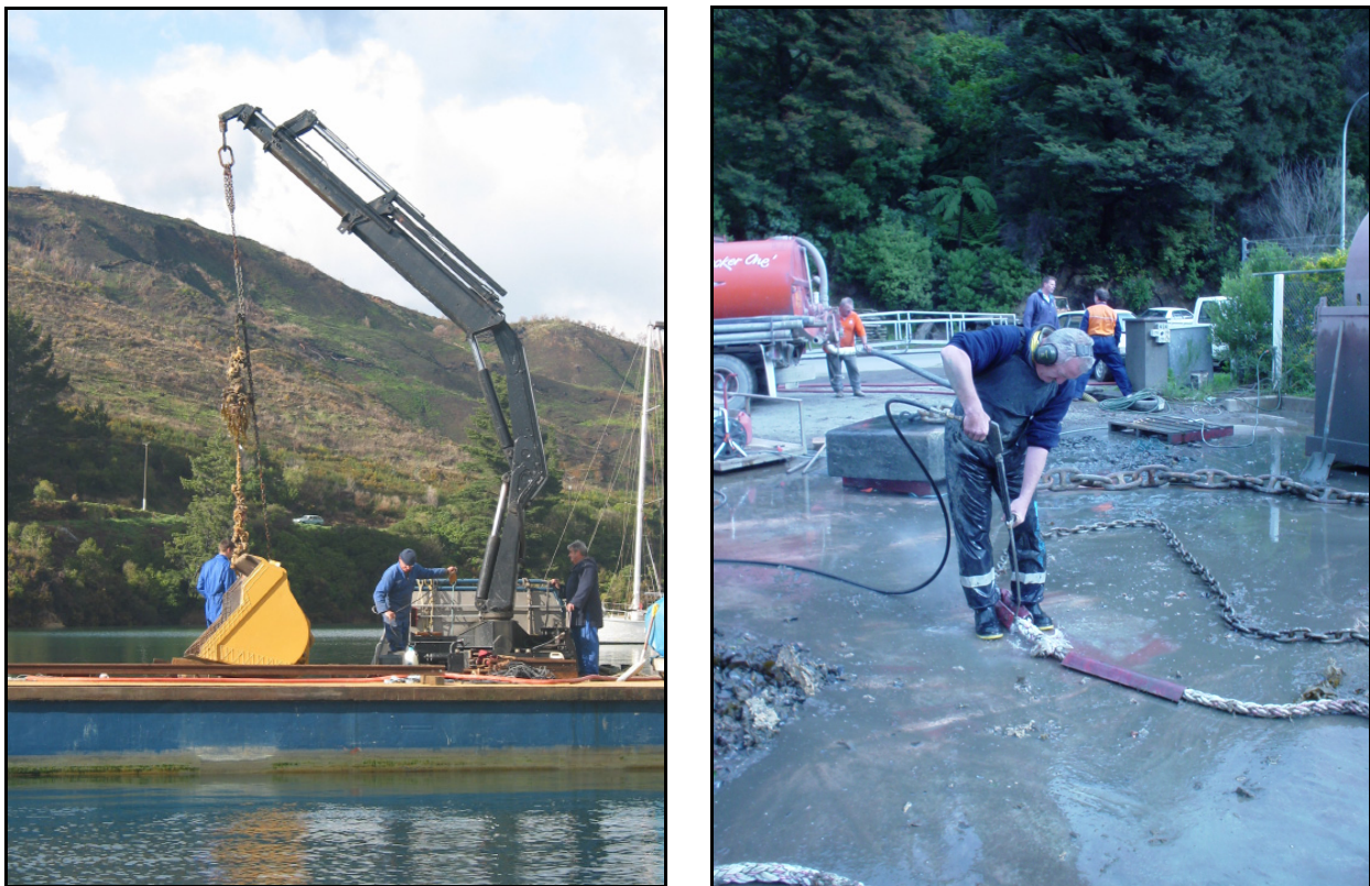
Figure 12. Infected moorings were removed from Shakespeare Bay, water-blasted in a biosecure area (see footnote 3 on previous page for definition) in Picton and returned 48 hours later.
