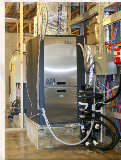
Ground source integrated heat pump
