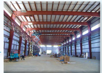
Inside Carbon Fiber Technology Facility production area.
