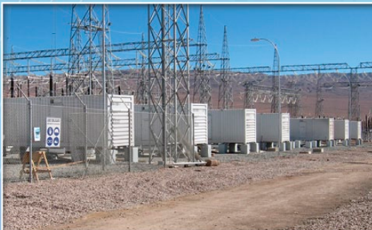
Lithium Ion Batteries (Image Courtesy of A123 Systems Smart Grid Stabilization System (SGSST™))
