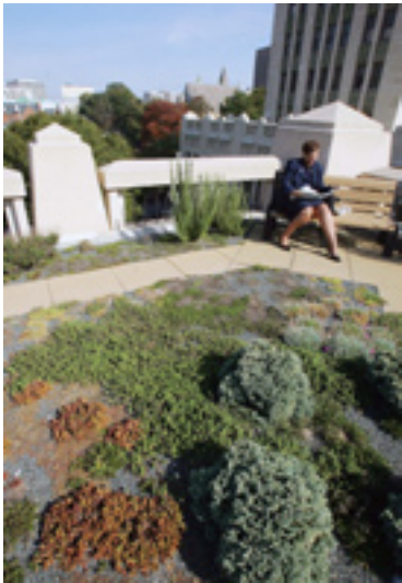
Green roofs, like this one in Atlanta, Georgia, are made of grasses and shrubbery and are designed to reduce energy use, filter pollutants from rainwater, and cool down cities during warm months.
