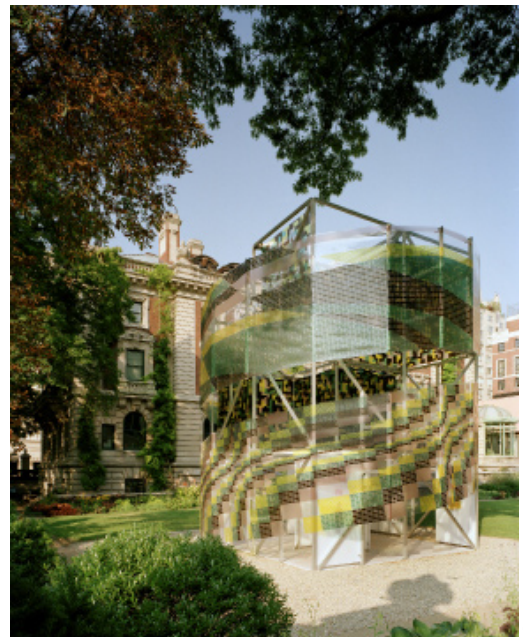
SmartWrap is a building material that can provide a structure with several functions, including climate control, lighting, and power.
