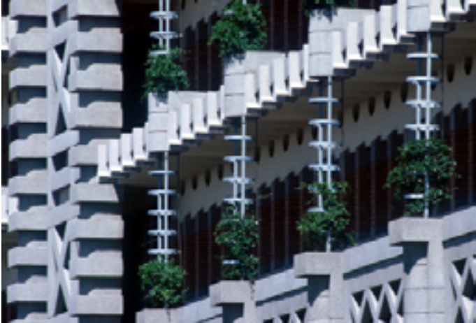
This building in Zimbabwe was designed to mimic a temperature efficient African termite mound, and reportedly uses 90 percent less energy than a conventional building.
