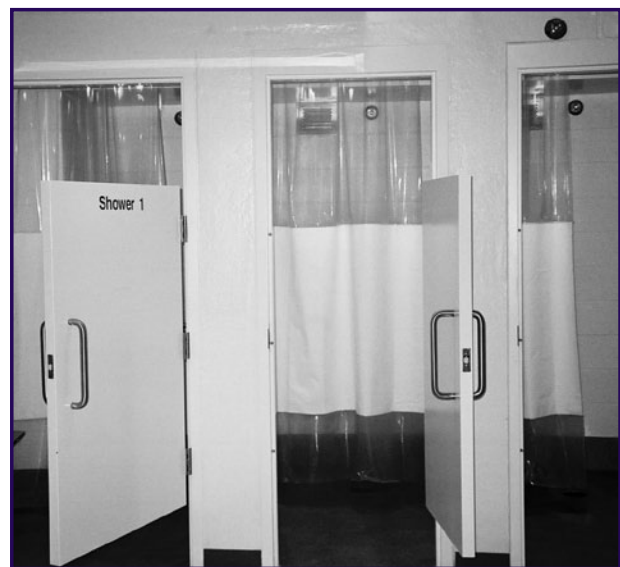
Showers in a housing area with both a door to the dressing area open at the top and bottom and a shower curtain that is clear at the top and bottom for the shower area.
