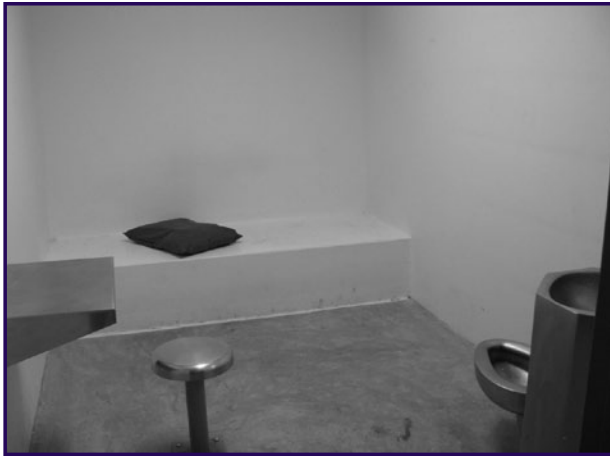
An austere disciplinary detention cell with concrete bunk (the mattress was temporarily removed from the cell), steel desk, food pass, and stainless steel combination fixture.
