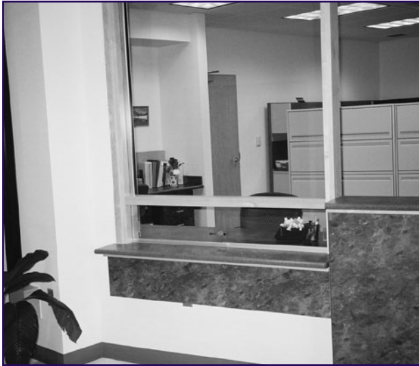
Receptionist's window with a sliding opening to receive items from the public. (Photograph courtesy of Voorhis Robertson Justice Services.)
