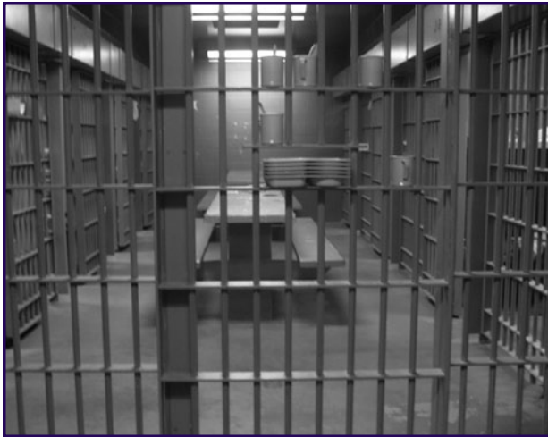
Poor sitelines in a linear-designed cell block. (Photograph courtesy of Jim Rowenhorst.)
