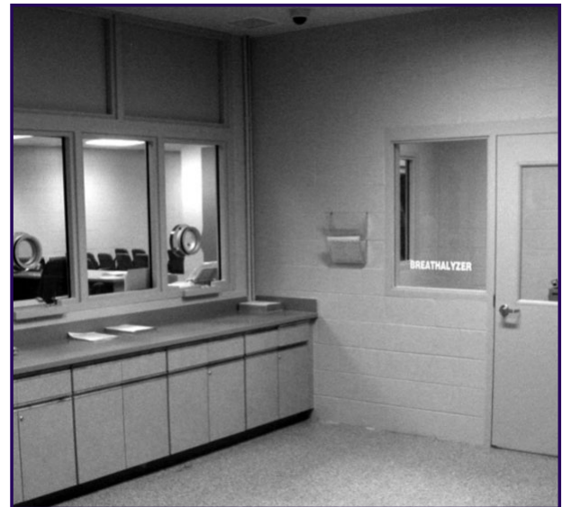
A room for breathalyzer equipment on the right that is accessible from within the arresting officer vestibule between the vehicle sallyport and the intake area. The intake area is beyond the glass on the left.
