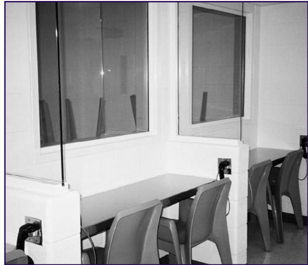
Open-backed visiting stations within one large enclosed visiting room, all with good visibility and easy accessibility. (Photograph courtesy of Liebert & Associates.)
