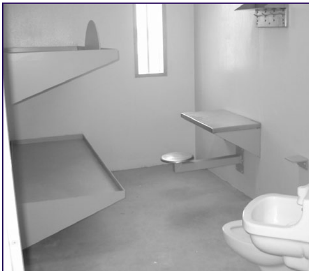
Double-occupancy cell in a direct supervision facility with fixed desk and porcelain fixtures.
