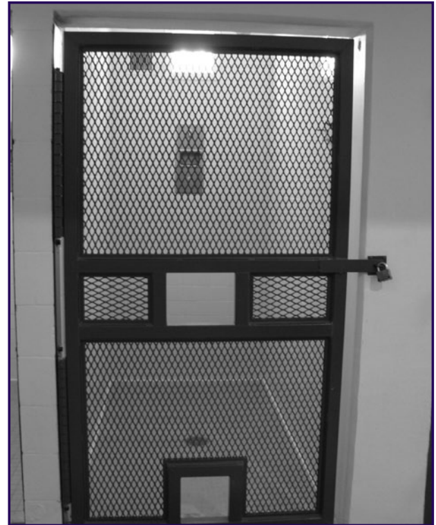
A secured shower in an administrative segregation unit. Note the ports used to remove restraints.
