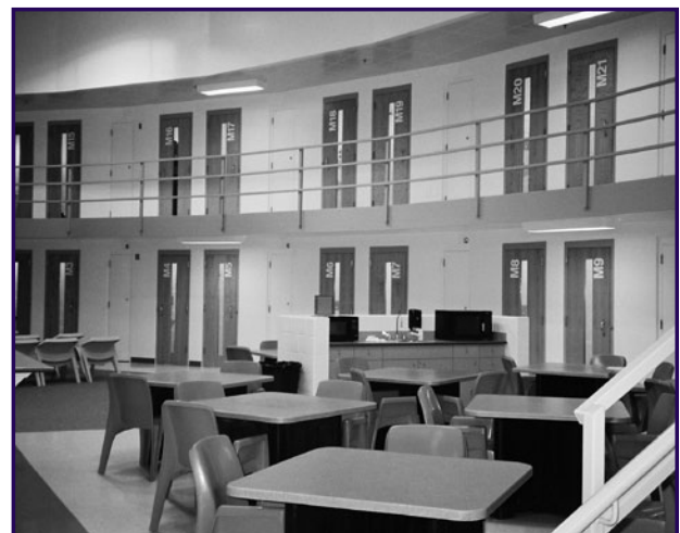
Housing unit within the secure perimeter and primary internal security zone with solid-core wood doors, nonfixed furnishings, and open officer's station.
