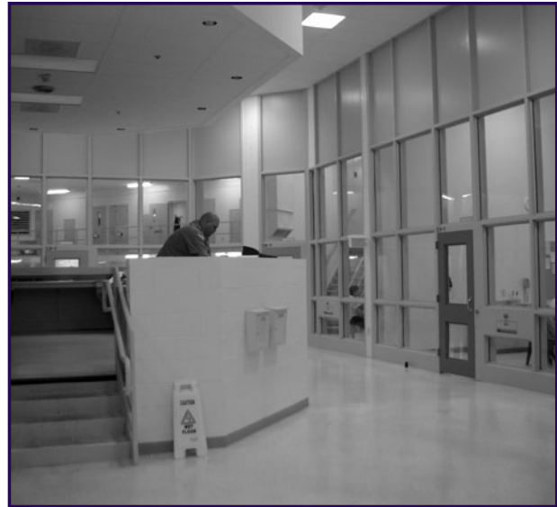
Open housing control booth with a good view of cell fronts, dayrooms, and mezzanine walkways.
