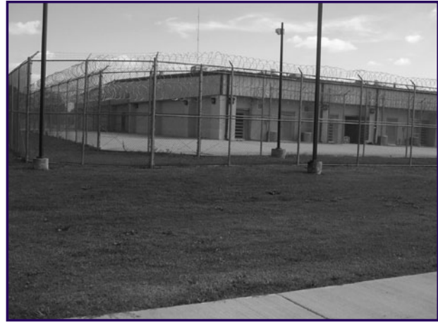
Jail with dual fenced perimeter with razor wire. (Photograph courtesy of Jim Rowenhorst.)
