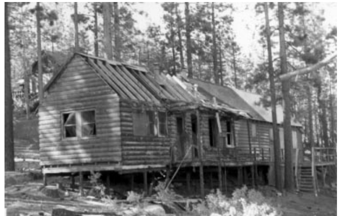
Building damaged in fire set by vandals. OIG photo.
