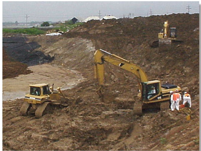
More than 80,000 cubic feet of soil was excavated to complete Phase 1.
