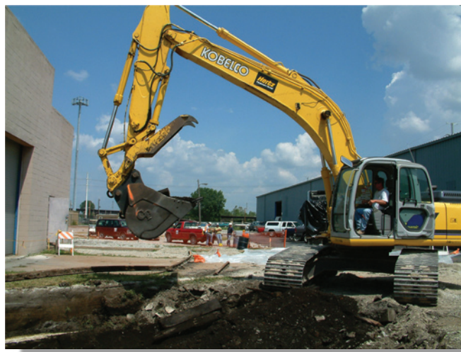
Excavation begins at Heintz Steel and Manufacturing.
