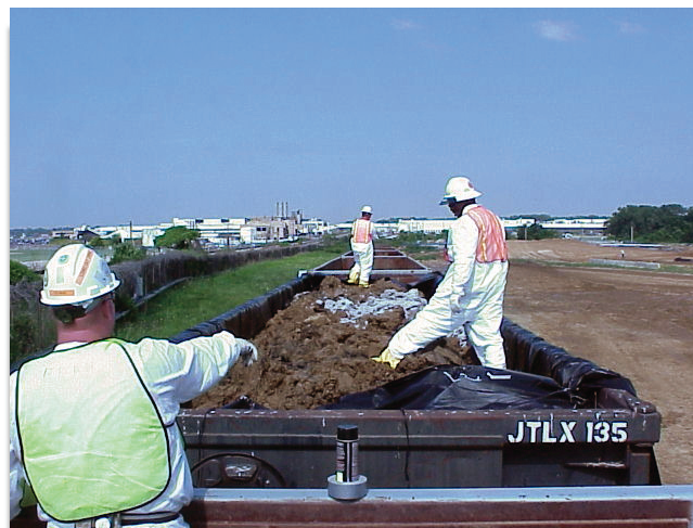
Crews prepare material for shipment from SLAPS.
