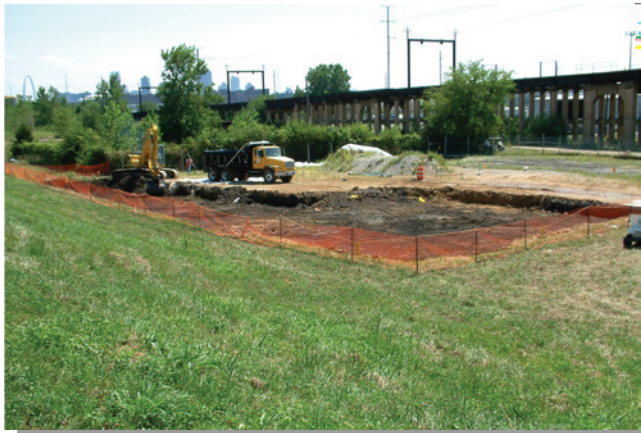
Crews are removing material from Plant 7 East.
