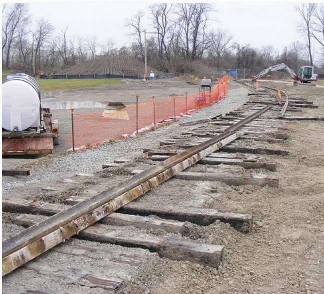
Removal of HISS Railspur
