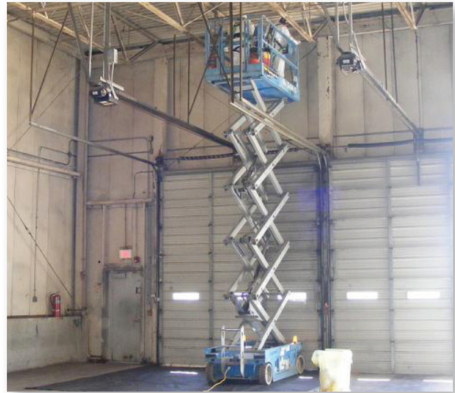
Decontamination of the building at VP 02(L)
