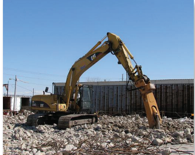
Demolition of SLDS 700 Pad
