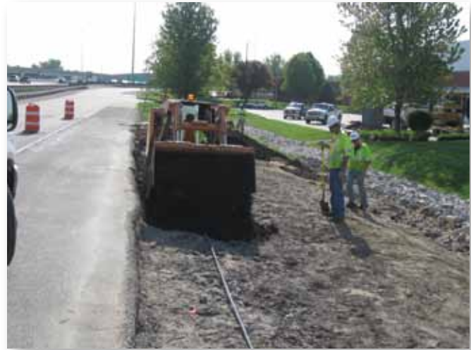
Restoration of VP-54 along Pershall Road
