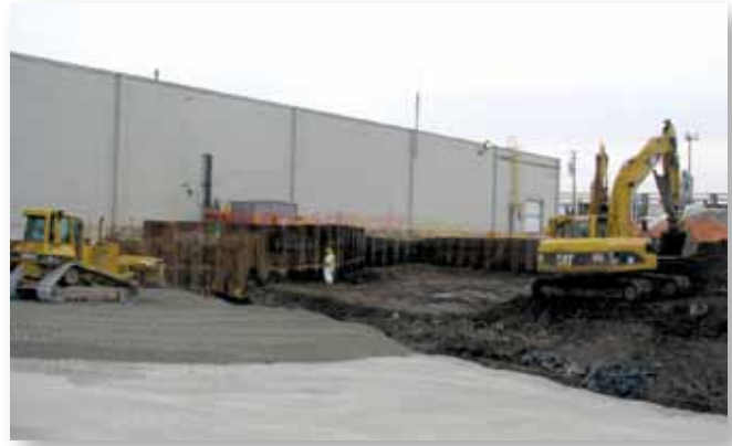
Plant 6-West Half Excavation
