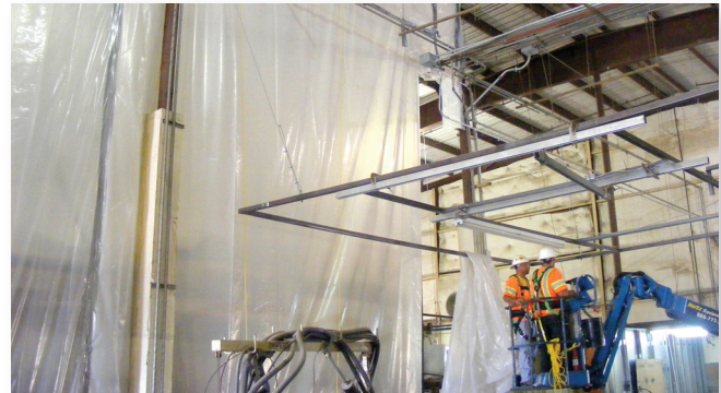
Futura Building 2/3 Decon Prep Work
