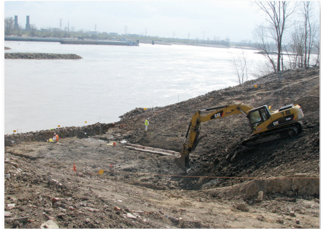
City Property Phase 2 (Area 7) Looking East
