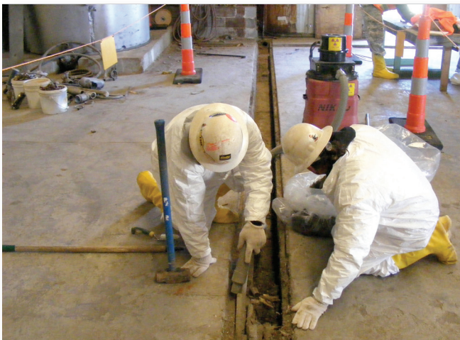
Futura Building 4 Raceway Decon
