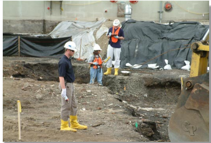
A five-year review will assess cleanup underway at the St. Louis Sites. Workers here take soil samples to monitor conditions as cleanup progresses.
