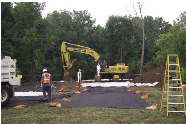
An estimated 950 cubic yards of contaminated material was removed from the Ballfields in September.
