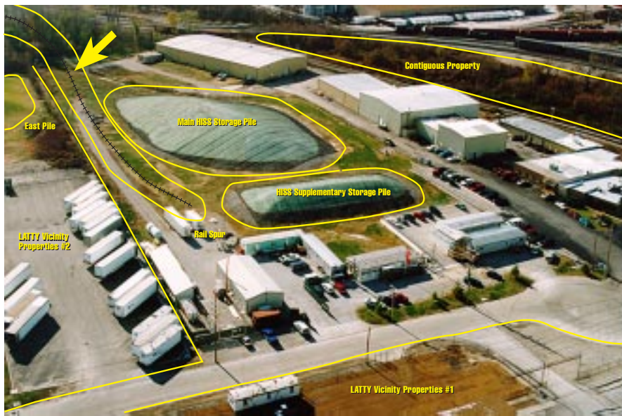
The HISS rail-loading facility is scheduled for completion and full operation in 1999.
