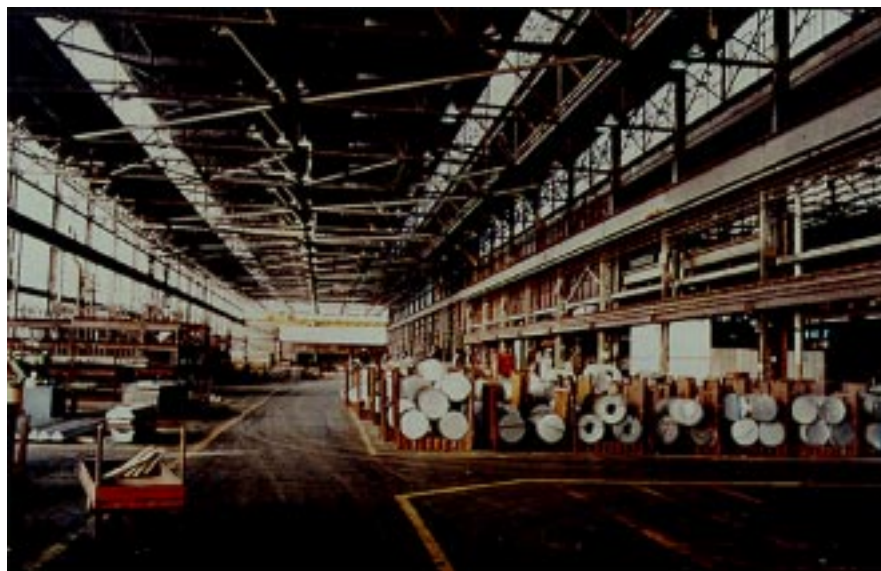
The Madison Site consists of two large, interconnected buildings of similar design and shape.
