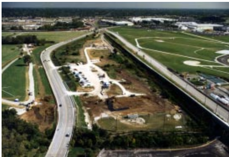
Aerial photograph of SLAPS and the North Ditch Area.
