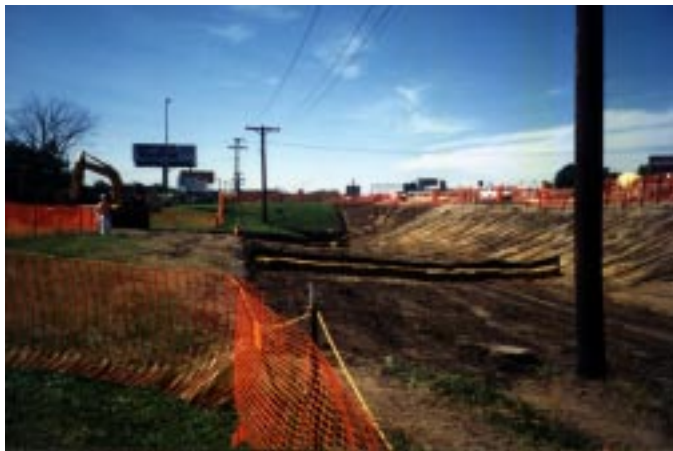
Erosion controls were used at VP 56 to prevent offsite flow of contaminated materials.
