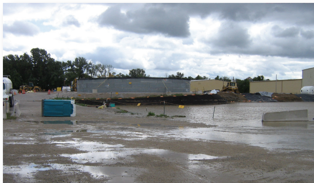
Flooding from Hurricane Ike caused extensive damage to storage buildings, their contents, and vehicles parked outside the buildings at the east end of HISS.
