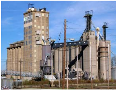
Cargill Grain Elevator
