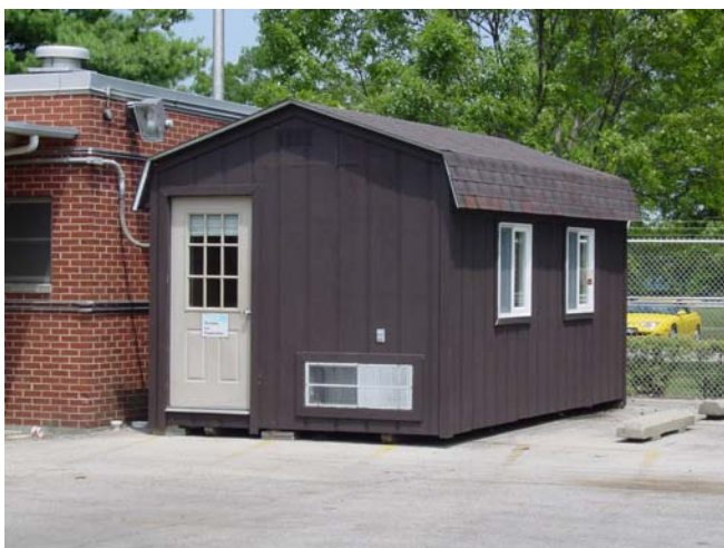
Portable building converted into office space
