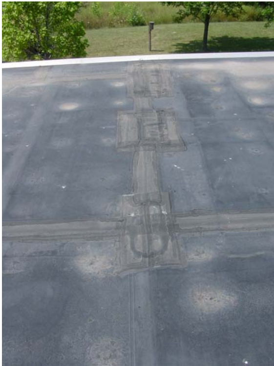
The roof has been patched in several places to stop it from leaking
