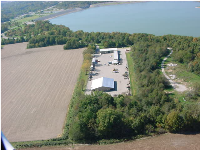
Arial photo of Maintenance Complex
