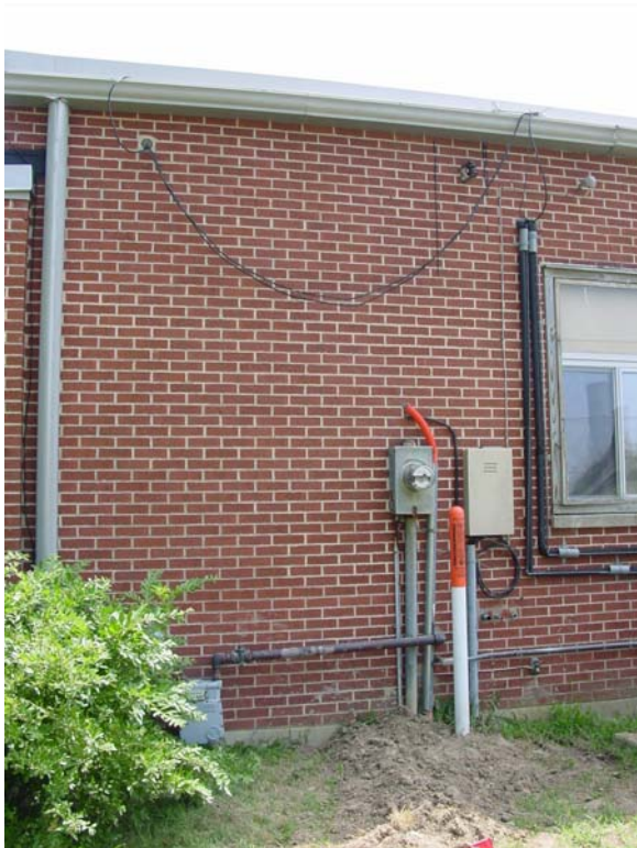
Existing wiring for electronic equipment and telephones does not have the capacity to provide the proper services needed
