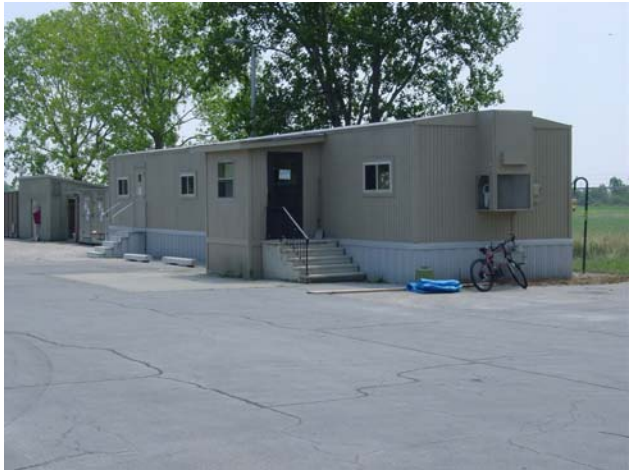
Trailer surplused from Carlyle Lake that serves as the Interpretive Services Office
