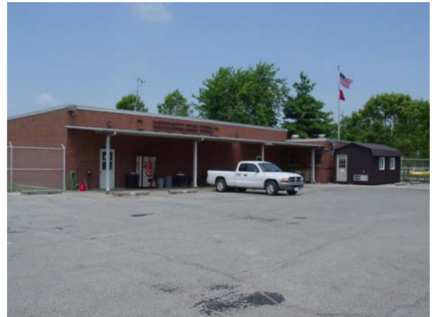
East side of the Administration Building
