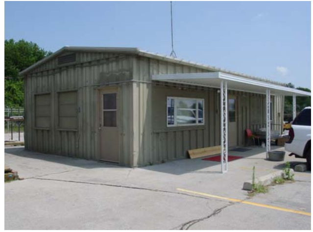
Salvaged Sewage Treatment Plant Building that serves as the Natural Resources Office
