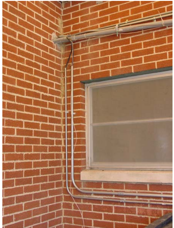
Existing wiring for electronic equipment and telephones does not have the capacity to provide the proper services needed
