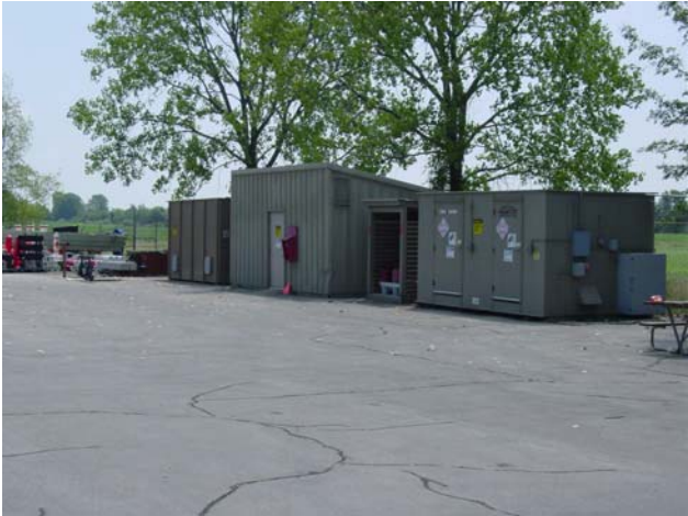
Chemical, power tool, paint, and oil storage sheds
