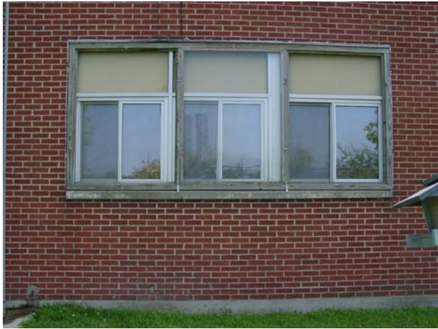
Makeshift Storm Window Frames had to be Installed
