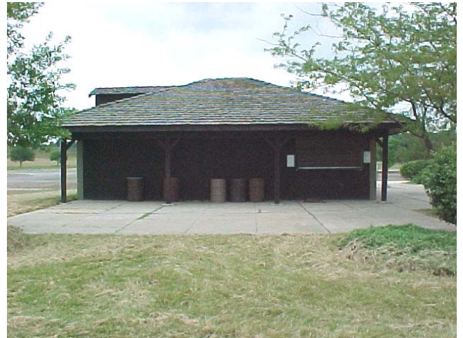
Rehabilitate Vending Area. Consession Building has been removed, provide vending hookups, and replace and relocate beach picnic shelter
