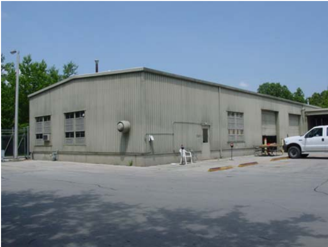
Building that provides maintenance work space
