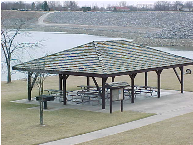
Install Electrical Services to the Overlook Berm Picnic Shelter
