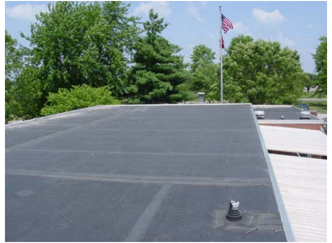
The roof on the Administration Building is a rubberized flat roof
