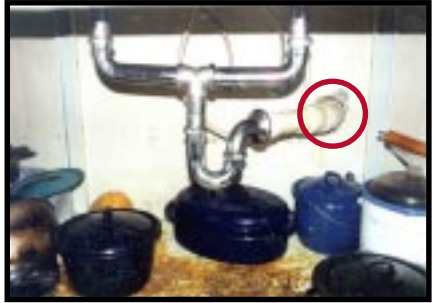
Look for gaps where the water pipes come into your home
