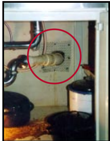
Use lath metal around pipes
