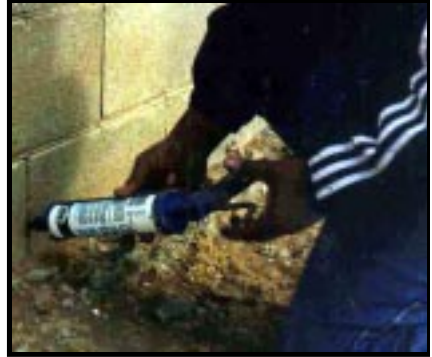
Seal holes with caulk
