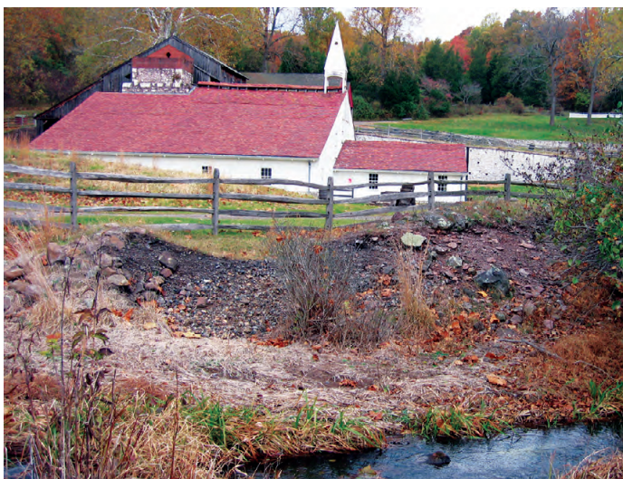
Figure 1. The cast house at Hopewell Furnace National Historic Site, Pennsylvania. The cast house encloses the furnace. The stone stack of the furnace is visible on the left side of the cast house. In the foreground, part of the furnace slag pile is exposed and makes up the left bank of French Creek.
