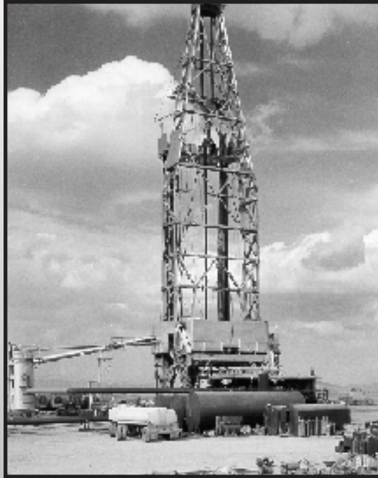
An Emsco 1500 heavy duty drilling rig is drilling an 64-inch 3,850 foot emplacement hole for the Jorum test which was detonated on September 16, 1969.
