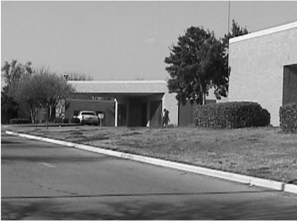
Fig. A.2.4. View of Regional Medical Center.
