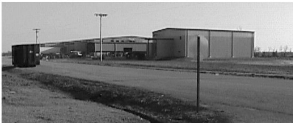
Fig. A.2.2. View of rebuilt plant.
