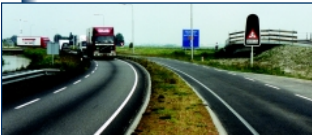
Figure 12. Narrow lane widths, The Netherlands.
