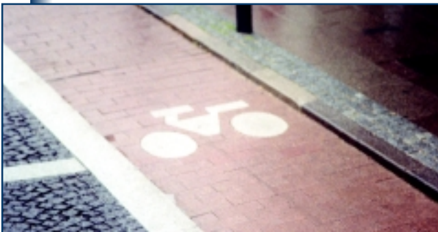
Figure 38. Bike lane separated with color coding, Denmark.
