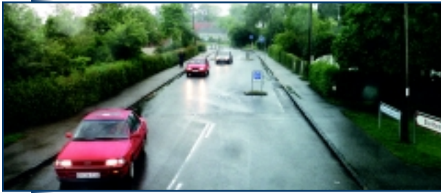
Figure 18. Narrowing with signs, Denmark.
