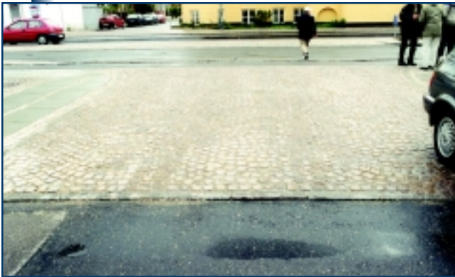
Figure 27. Table with different pavement texture, Denmark.
