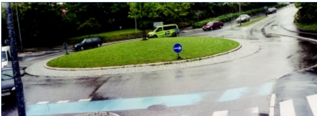
Figure 44. Bike path sharing the roadway, but color coded, Denmark.
