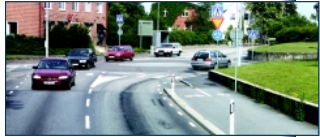
Figure 22. Small roundabout flush with pavement, Sweden.
