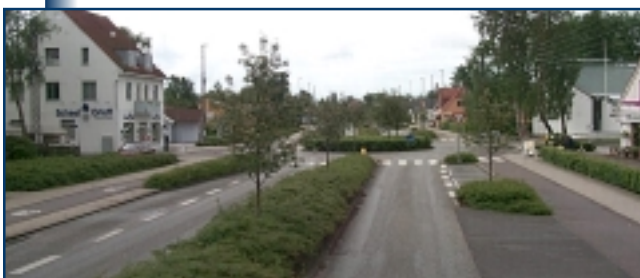
Figure 21. Combination of several traffic calming elements: islands, roundabout, and narrow lanes, Denmark.
