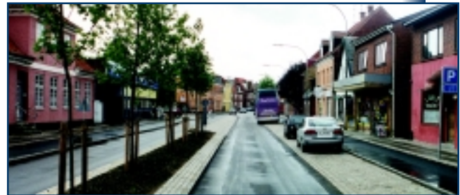
Figure 23. Combination of several traffic calming elements: islands, narrow lanes, and pavement textures, Denmark.
