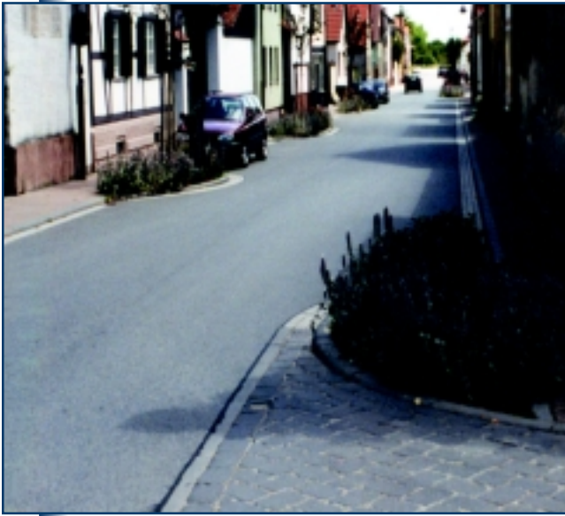
Figure 26. Chicane and pavement texture, Germany.
