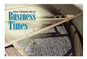
Contaminant floating on water in the dissolved air-flotation-tank (at lower right). Dissolved air forms bubbles that capture and lift free-product contaminant to the surface of the separator.
