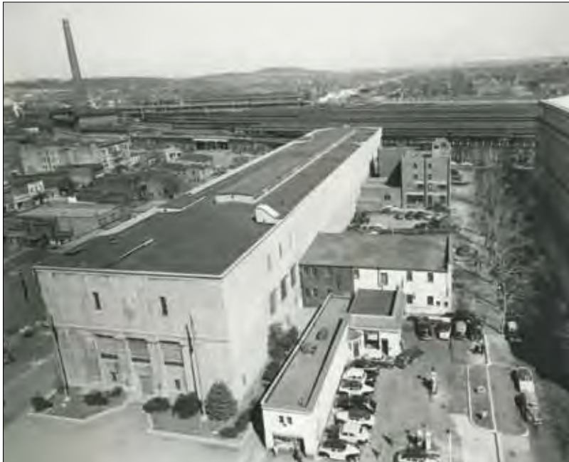
Building 4, on the east side of North Capitol Street between G Street and G Place NE. The building connects directly with the railroad by a bridge at the rear over 1st Street NE.
