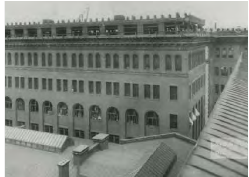
Among Public Printer Carter's first actions was the reconstruction of the top story of Building 1 to create new space, most of it devoted to "employee rest and recreation."
