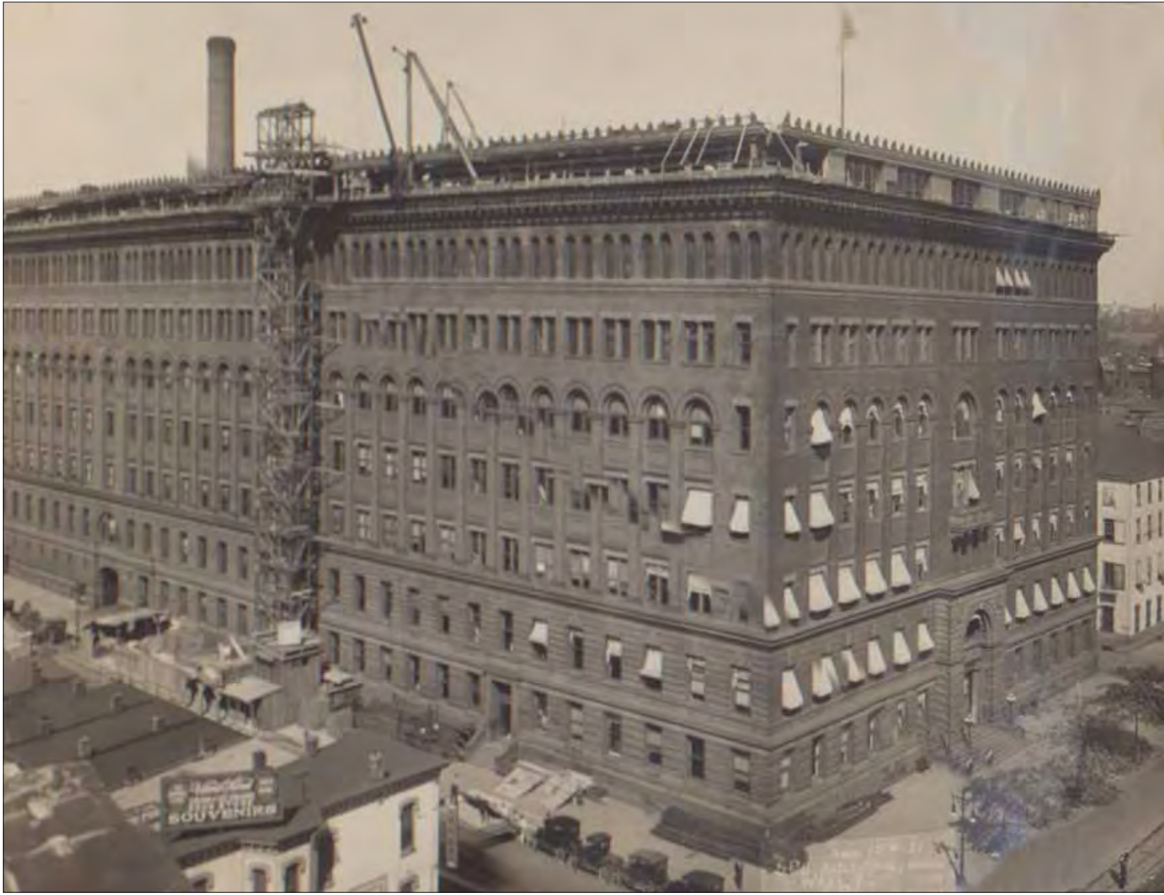
The renovations created a full eighth story with a cafeteria, auditorium, employee lounge, and bowling alley, as well as a new photoengraving plant and storage.
