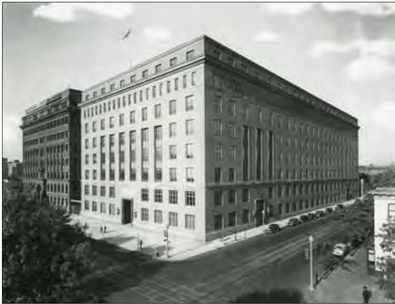
Building 3 at its completion in 1940.
