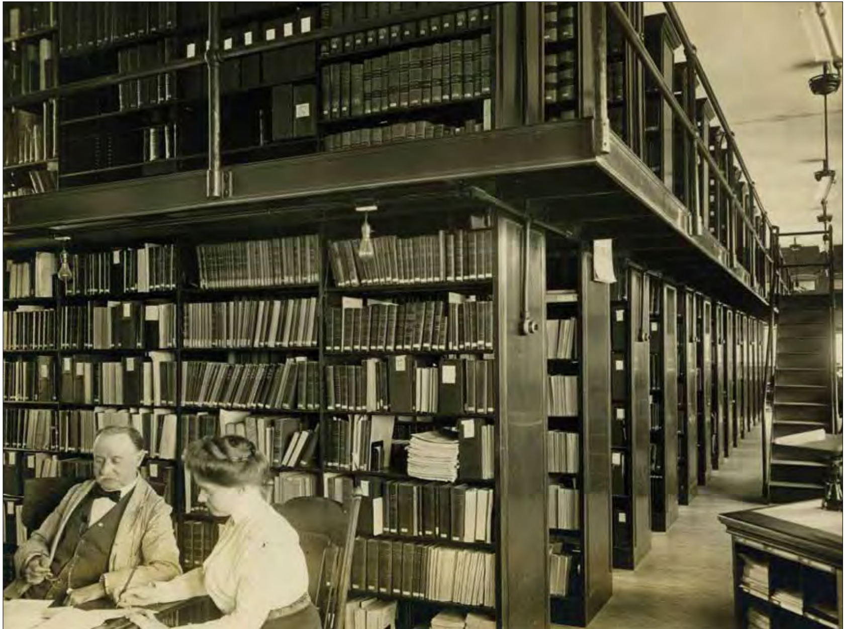
The Public Documents Library in the early years of the 20th century, after the Public Documents Division moved from leased space into the seven-story annex at the rear of the North Capitol and H Street site. The two-tier iron and steel book stacks were the latest in library design.
