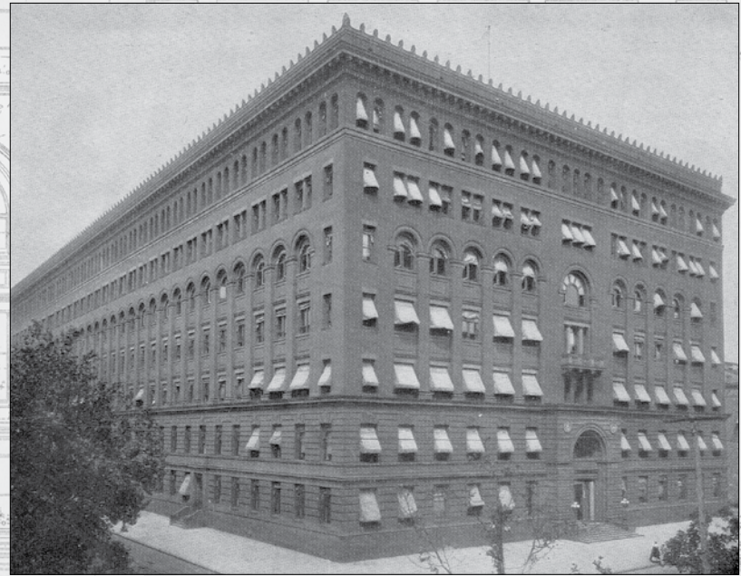
Building 1 soon after its completion in 1903. The most prominent image of GPO from Capitol Hill.
