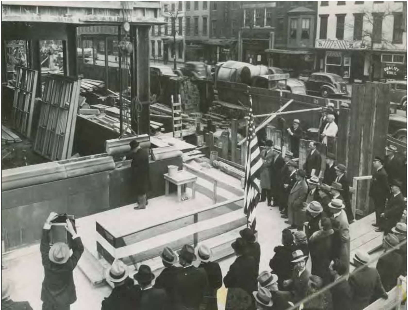
Public Printer Giegengack lays the cornerstone for Building 3 at the corner of North Capitol and H Streets NW, February 1939.
