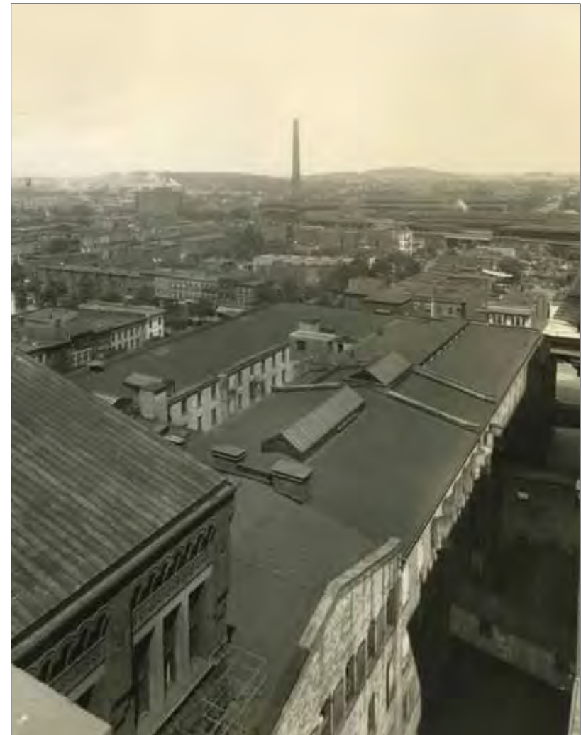
Giegengack successfully petitioned Congress to raze the grab bag of structures that had grown up around the original Wendell building. This photo overlooks the H Street site, probably from the 8th floor of Building 2.
