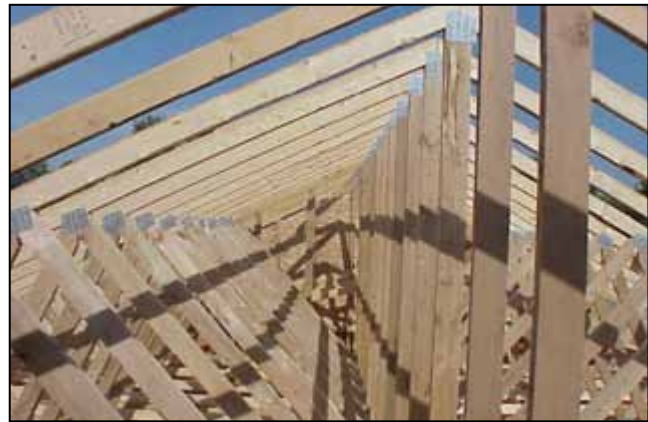
Figure 3.33. ~ Roof trusses containing hardwood lumber web stock.
