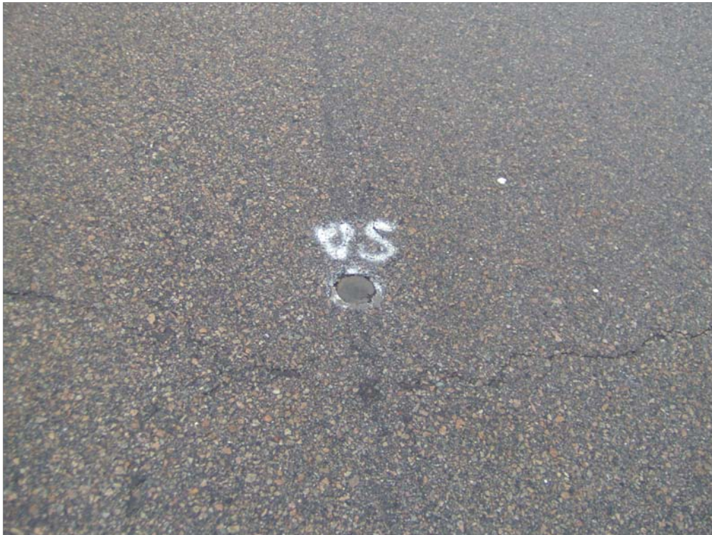
Figure 3. VDU Installed in Roadway
