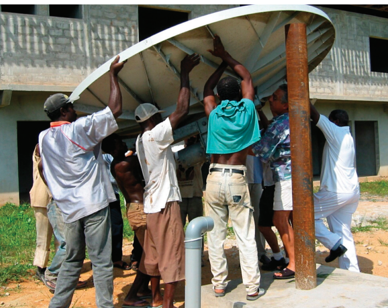
Installing the satellite dish for the Multilateral Initiative on Malaria communication network in Gabon.
