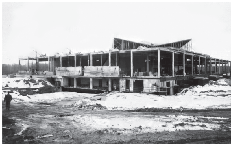
NLM Construction c. 1955
