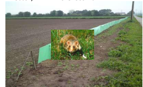
Site protection fence for endangered hamsters
