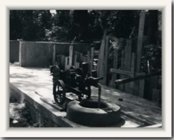
Construction of 20,000 gallon reservoir for storage of spring water
