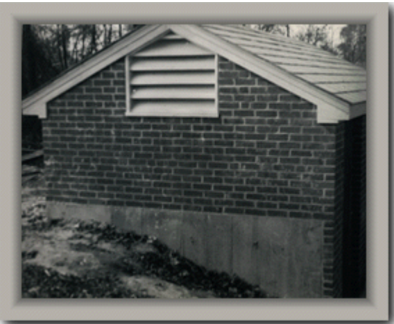
Pump house for spring reservoir
