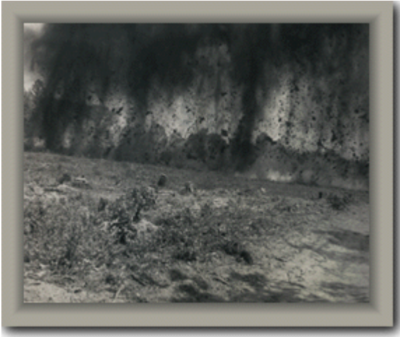
Dynamiting sluice-way drainage ditch for Cash Lake
