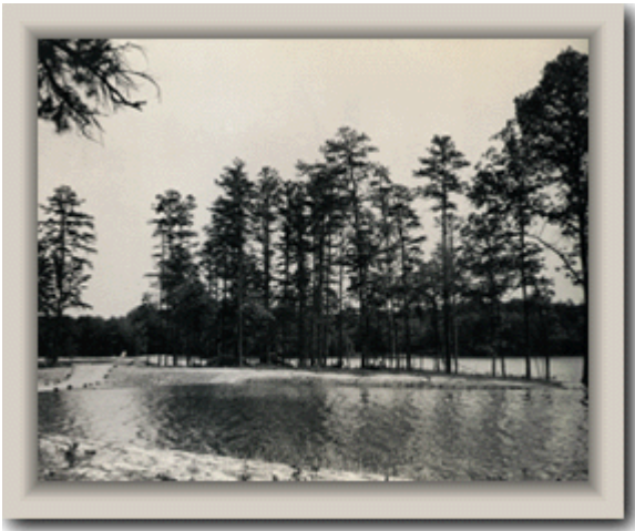
Cash Lake and dam from the spillway
