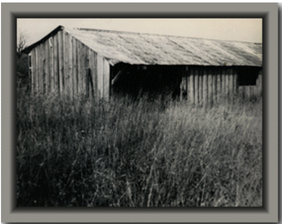
Shed for cattle and sheep razed in connection with the construction program
