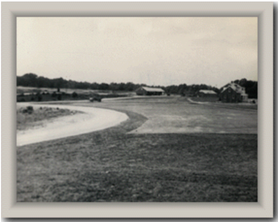
View from Snowden Hall looking toward garages
