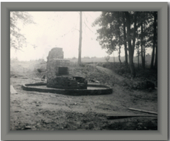
Picnic ground grille and oven prior to construction of shelter house
