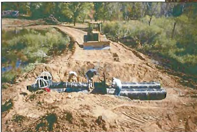
Water control structure construction, part of wetland restoration (bottom), and restored wetland (top), Kummer Landfill Superfund Case, Minnesota.
