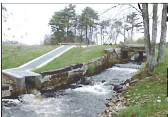
Fishway to restore passage for migratory fish, New Bedford Harbor Superfund Case, Massachusetts.
