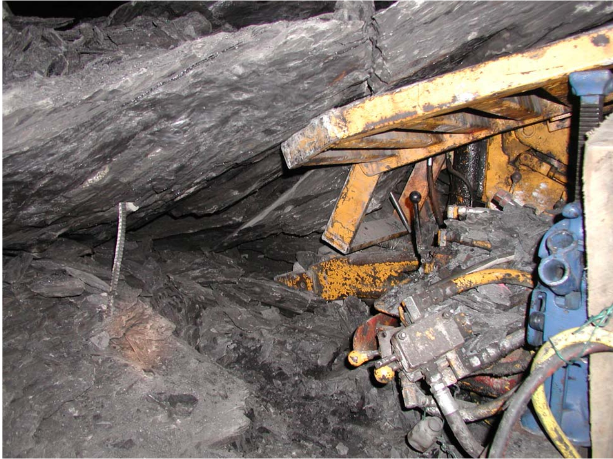
Photograph of Accident Scene Showing Galis 320 Roof Bolting Machine
