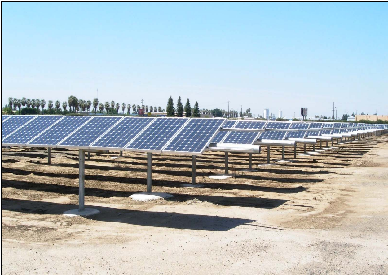
Figure 7: Example of a Ground-Mounted Solar PV Installation
