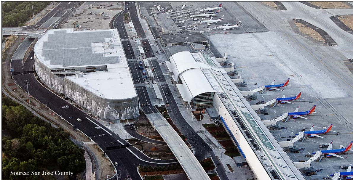
Figure 22: Solar on New Rental Car Parking Facility at Mineta San Jose Airport
