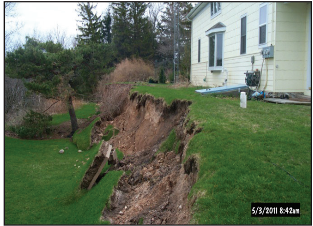
Bluff erosion threatens property and homes in the Great Lakes.
