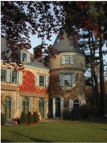
Grey Towers, Milford, Pennsylvania
