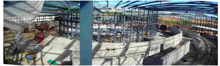
Tunnel. Picture: October 1 st 2007
