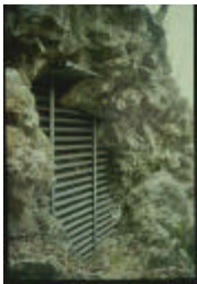
Bat gate installed in portal of Monte Cristo Mine, Rush Historic Mining District. Buffalo National River, Arkansas
