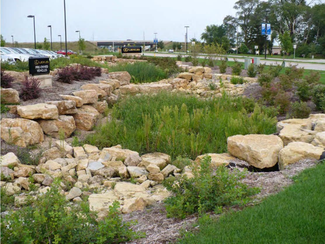
Figure 4. Infiltration basin at retail dealership on Airport Road in Middleton, Wis., in 2008. (Photo by W.A. Gebert)
