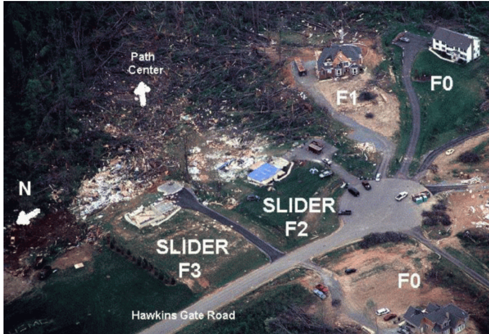
Photo 5. Aerial view looking east of residential damage at end of Hawkins Gate Road, located just east of La Plata, Maryland. Split-level homes slid off their foundations into a ravine. The home had been anchor-bolted to its foundation but failed where the wall studs were straight nailed to the bottom plate. (Courtesy of Tim Marshall, Haag Engineering)
